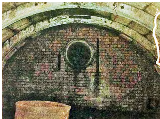
The tunnel before infilling with gravel in 2013
